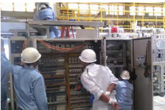
Electrical Wiring Work 1
