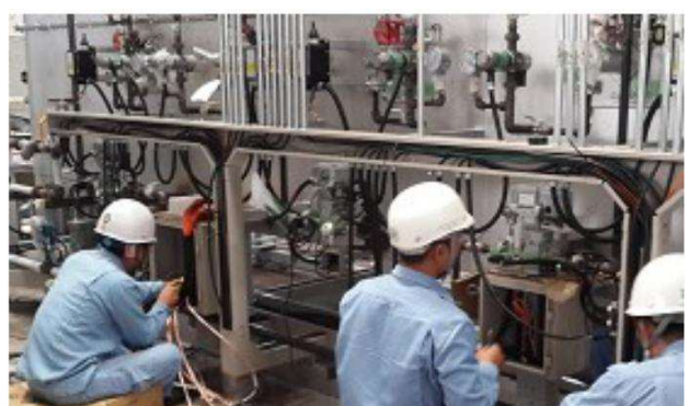
Electrical Wiring Work 2
