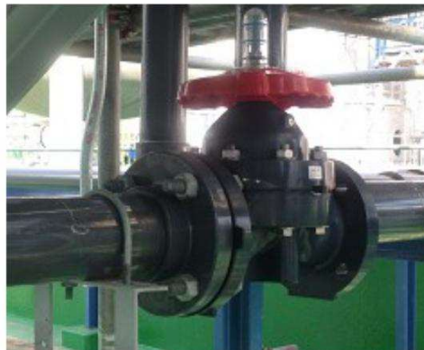
Change piping of Tank 2
