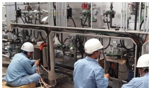
Electrical Wiring Work 2
