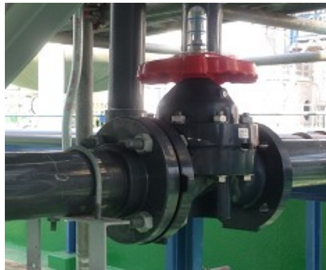
Change piping of Tank 2
