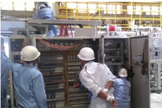
Electrical Wiring Work 1
