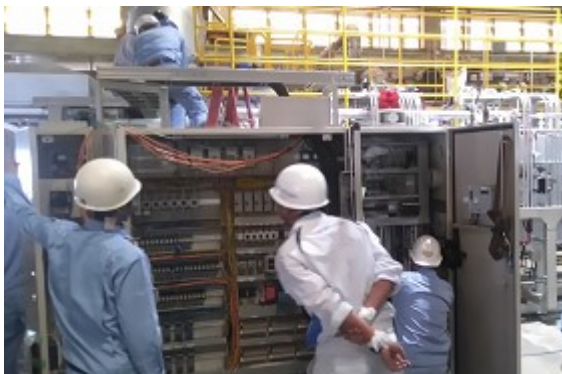
Electrical Wiring Work 1
