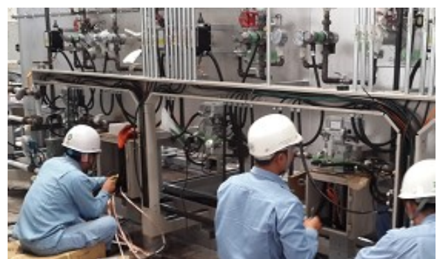
Electrical Wiring Work 2
