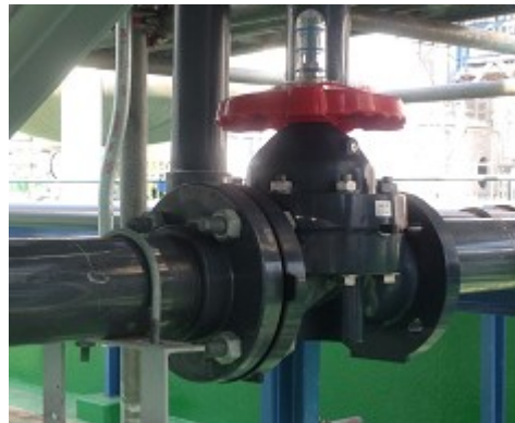
Change piping of Tank 2
